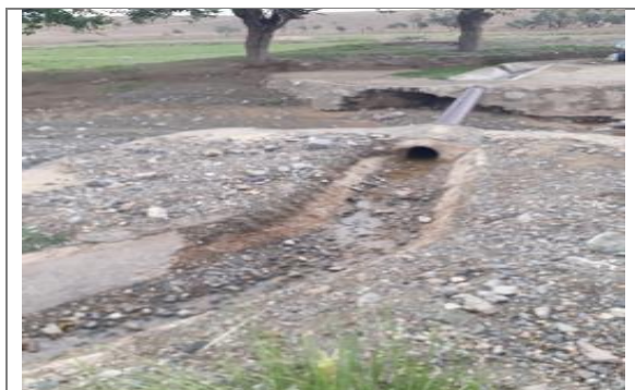
View of damaged PVC Pipe and Watercourse, District Kharan
