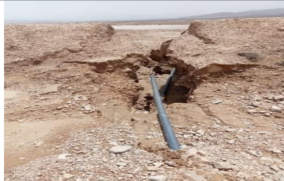
View of damaged Culvert, Watercourse and PVC Pipe, District Pishin
