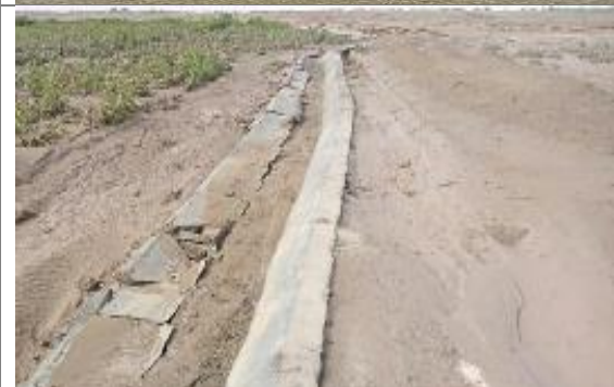
View of damaged PVC Pipe and Watercourse, District Kharan
